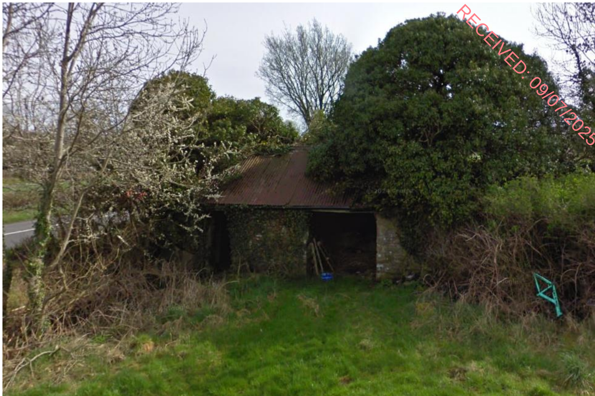
Figure 2.8 Structure to be demolished (Source: Google)
